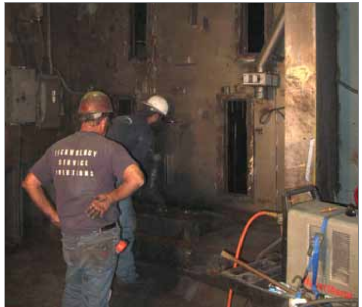
Install of 8 Wheel Rebuild
